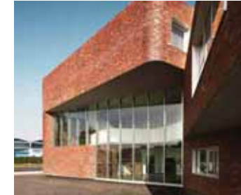
Brick and Glass Facade
